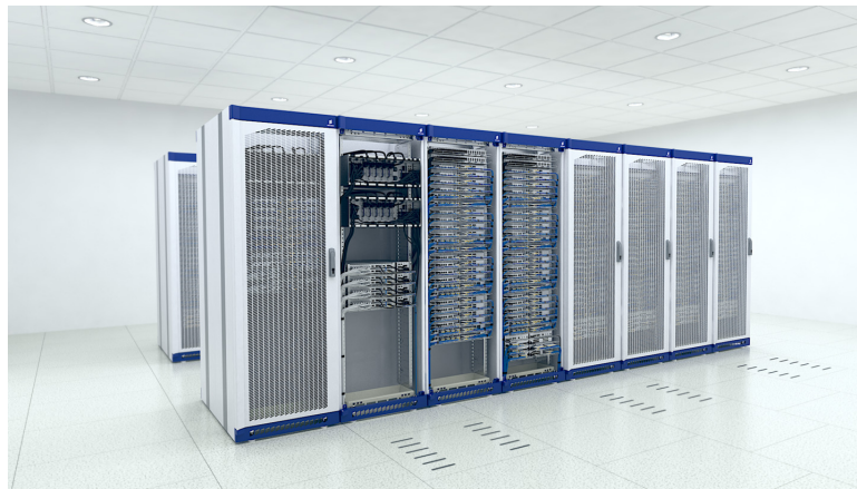
Figure 2.5: Several interconnected cabinets construct a large-scale telecommunication system. One node in Figure 2.3 can vary in size from a single circuit board up to several cabinets. Courtesy of Ericsson 2016.
